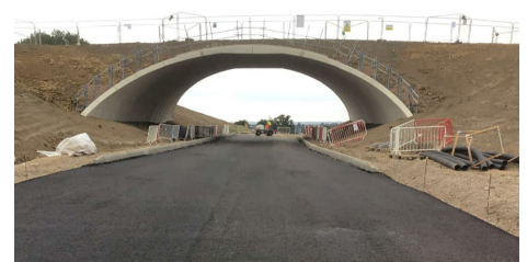
New asphalt laid under the green bridge
