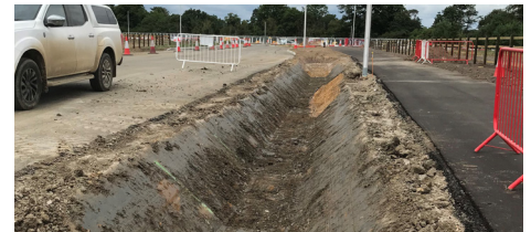
Works to the drainage swale
