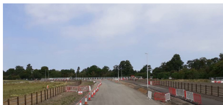
New street lighting columns erected at Bridge Farm roundabout
