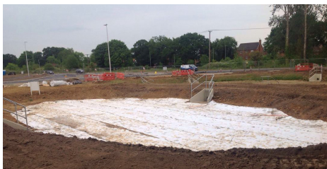
Pond liner installed within pond 3 at Duck Nest Farm roundabout
